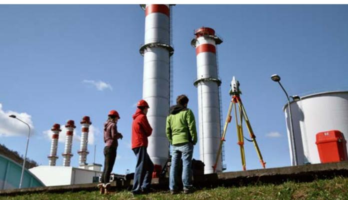
Laser scanning of tall chimney for determination of its non-verticality using modern total station
